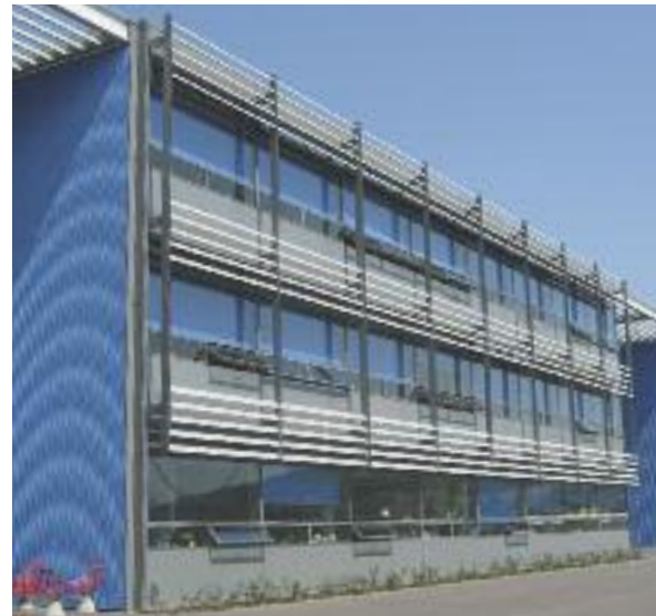
The Folkestone Academy in Kent was fitted with 400mm and 200mm wide Aerofoil Fins.
