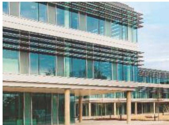
400mm wide fabricated, perforated Aerofoil Fins installed at the HQ of NAPP Pharmaceutical in Cambridge.
