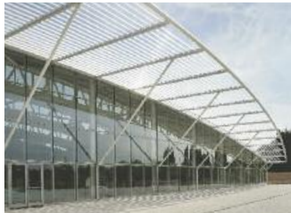
300mm wide extruded Aerofoil Fins installed as a horizontal canopy at Lee Valley National Athletics Centre in London.
