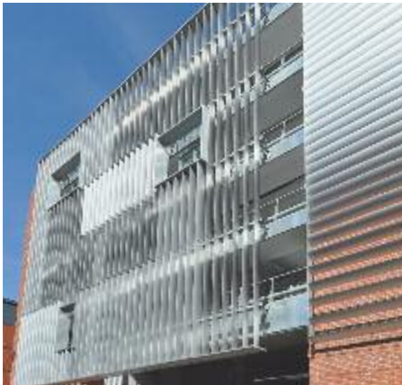
300mm and 450mm wide Aerofoil Fins installed at Q-Park as part of the Liverpool One development.
