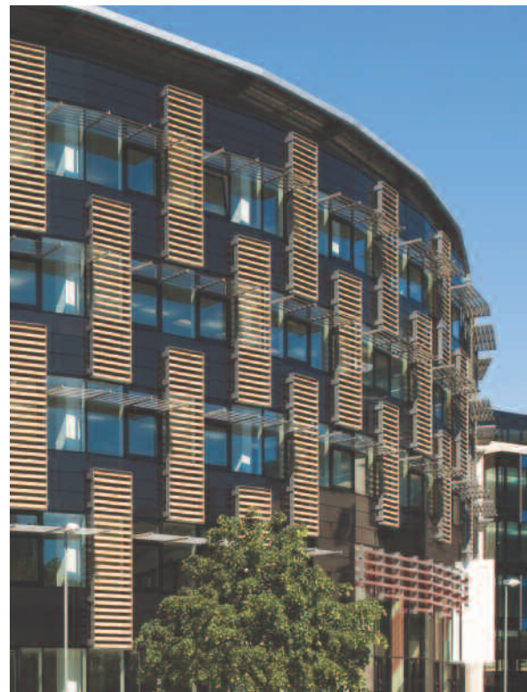
Levolux Timber Fins, Matrix XL and Glass Fins, secured using the Trinitix bracket at Exchange Place, Edinburgh. This helped the building achieve a BREEAM 'Excellent rating'.
